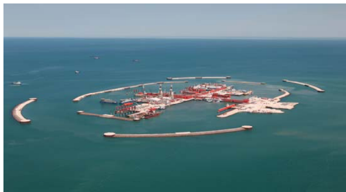
AGIP KCO's Kashagan Oilfield Offshore Island Project in the Caspian Sea. This photograph shows an artist's impression of the offshore artificial islands and barges. The design includes building production hubs on platforms and artificial islands to collect production.
